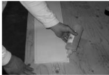
13) Apply adhesive to final panel
