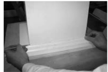
18) Use column shaft to mark cut lines for miters (cut long and work your way shorter for best results)
