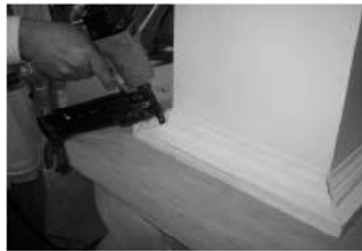
19) Apply adhesive to moulding and pin-nail into place.
