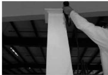
16) Glue ¼ cap piece and slide into place. Pin nail cap moulding to top of column.*
