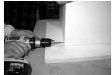
15) Screw or nail final panel to secure
